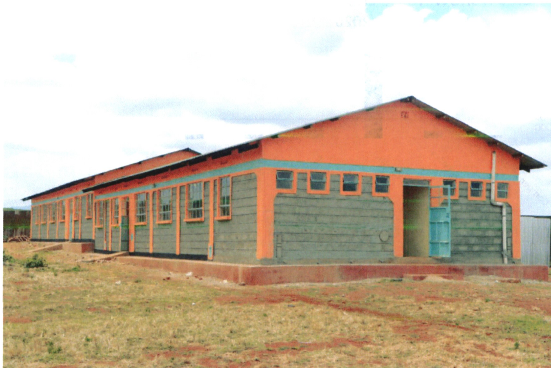
Figure 1: Girls Dormitory at Japata Secondary School
