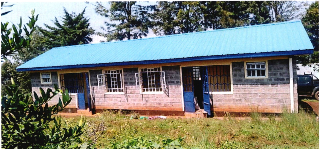
Construction of two units staff houses at Twendane Primary school
