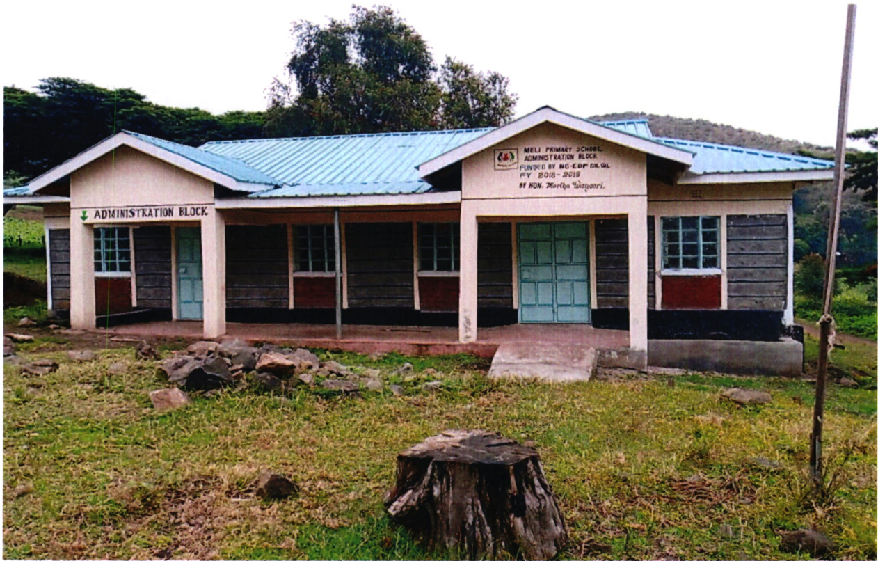
Construction of an Administration house at Meli Primary school
