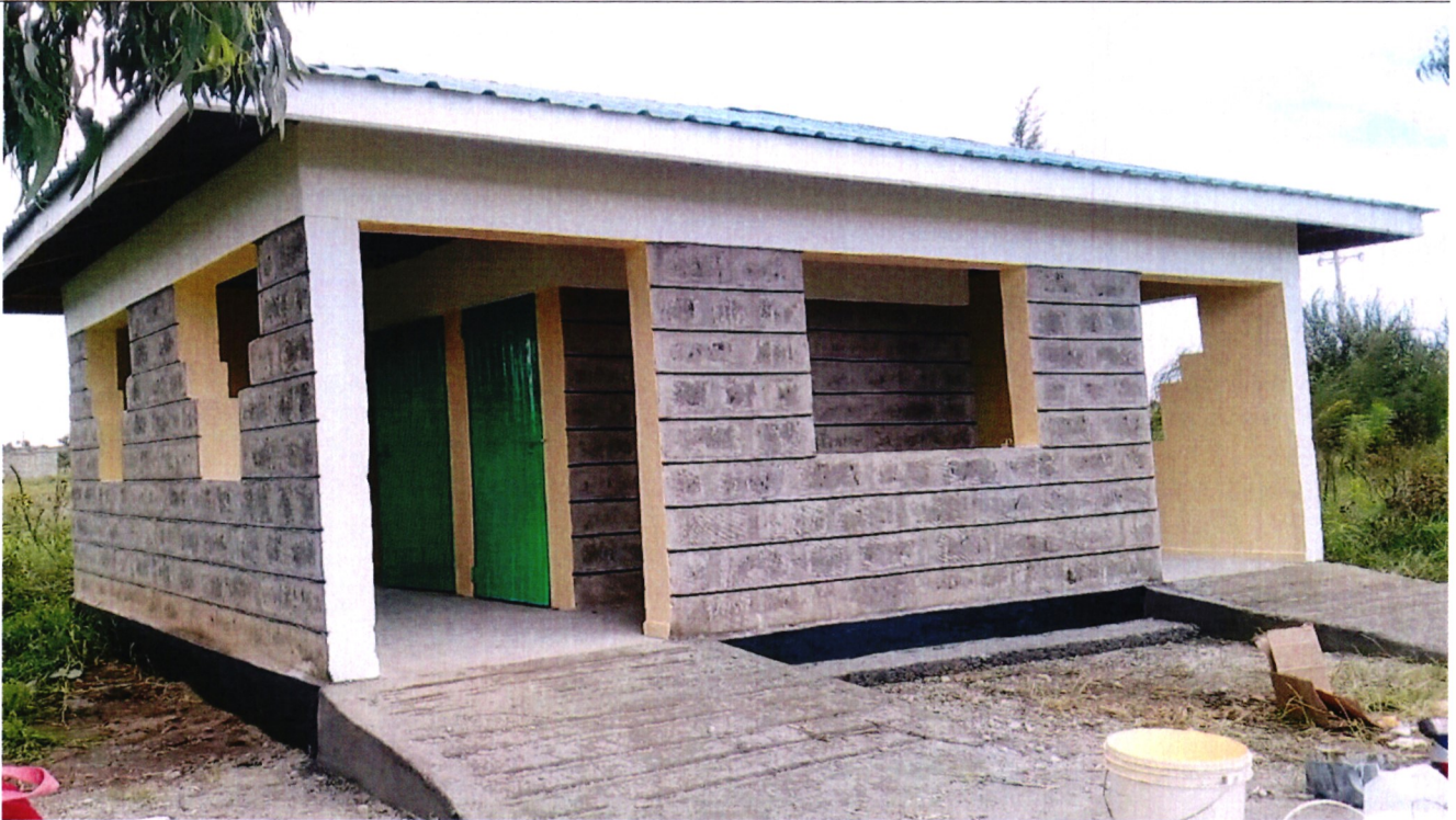
Construction of a six door pit latrine at Mwega Primary school
