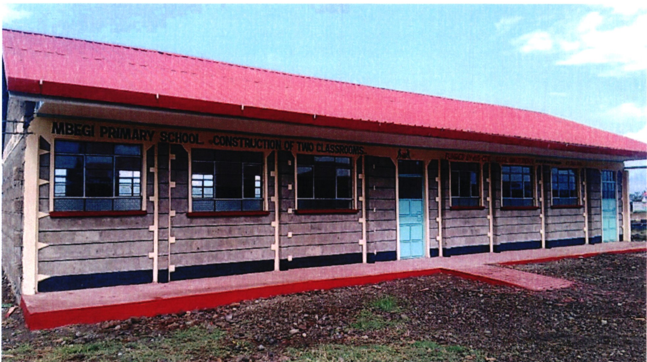
Construction of two classrooms at Mbegi Primary school
