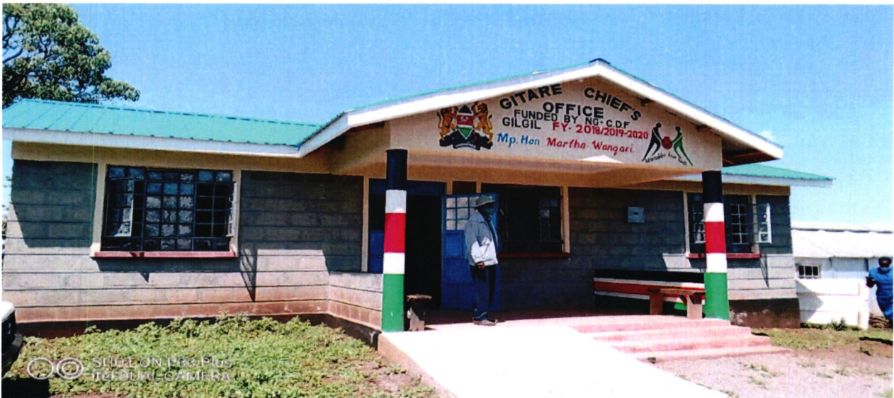
Construction of a Gitare Chief's offi
