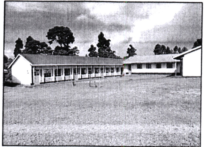
Makhonge Primary School (8 Classrooms)
