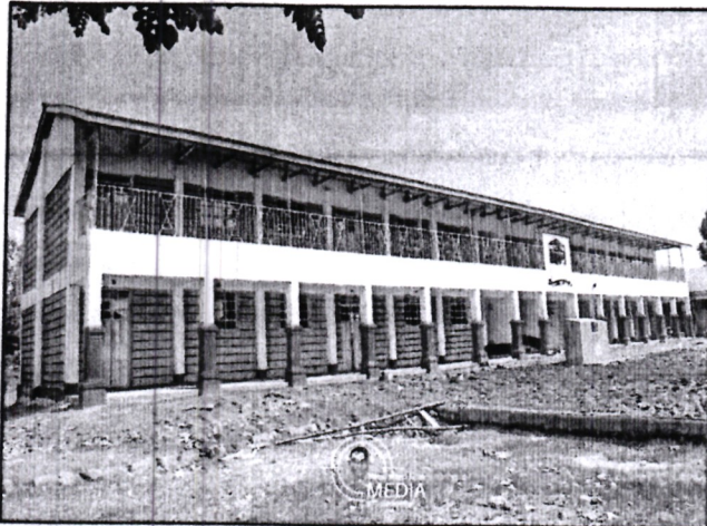
Matili Primary Schools (8 Classrooms Storey)
