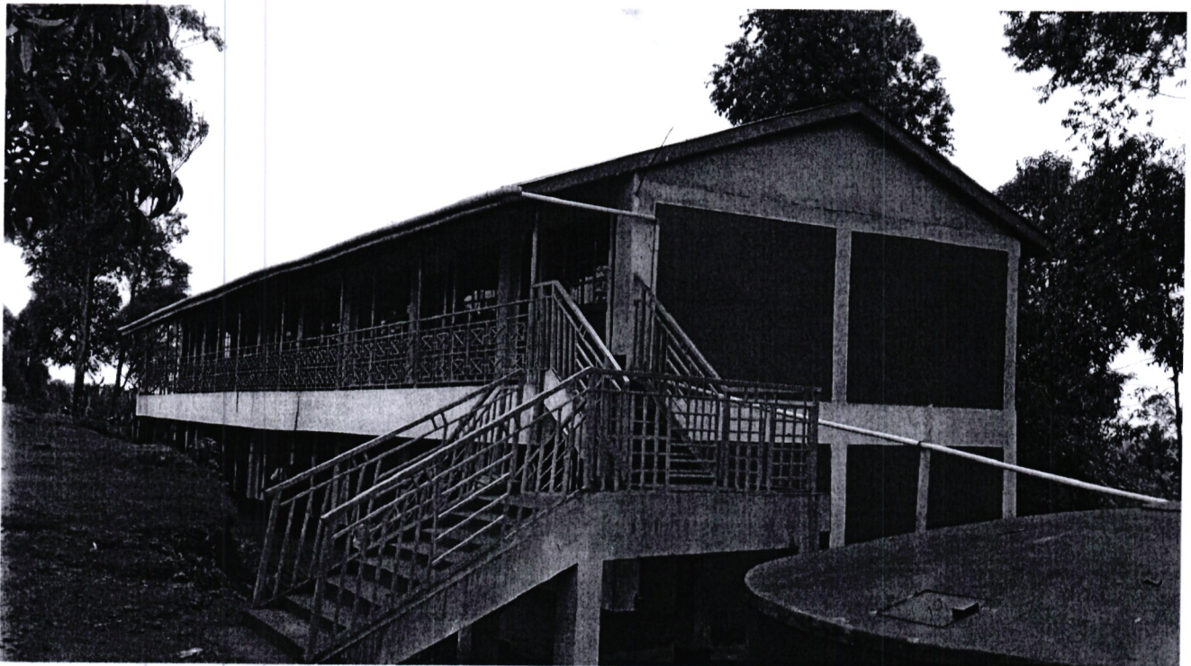
KITUTU CHACHE SOUTH NG CDF PROJECT-8 CLASSROOMS CONSTRUCTED BY NG-CDF AT KIANYABINGE PRIMARY SCHOOL
