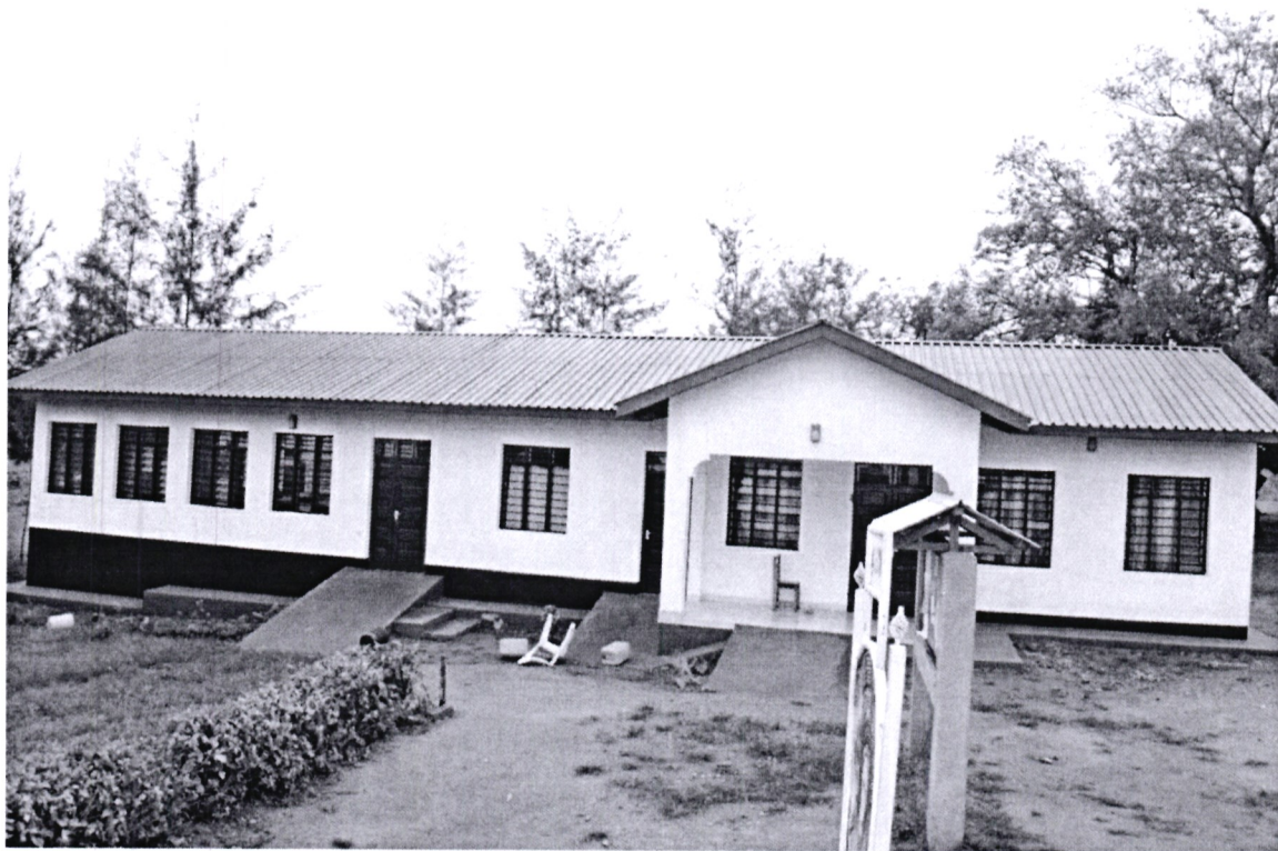
Mwenza mwenye Secondary School administration block
