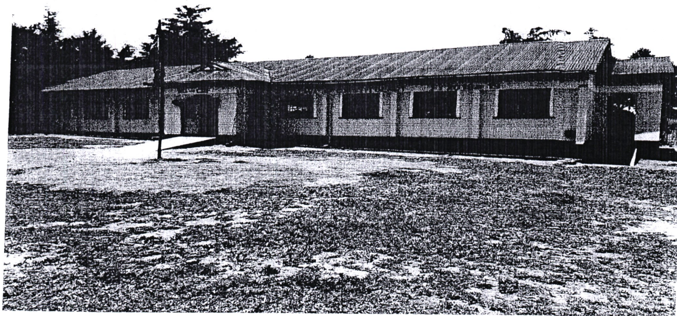
Silungai Boys High School construction of Dormitory funded by Malava NGCDF Financial Year 2018/2019 and 2019/2020
