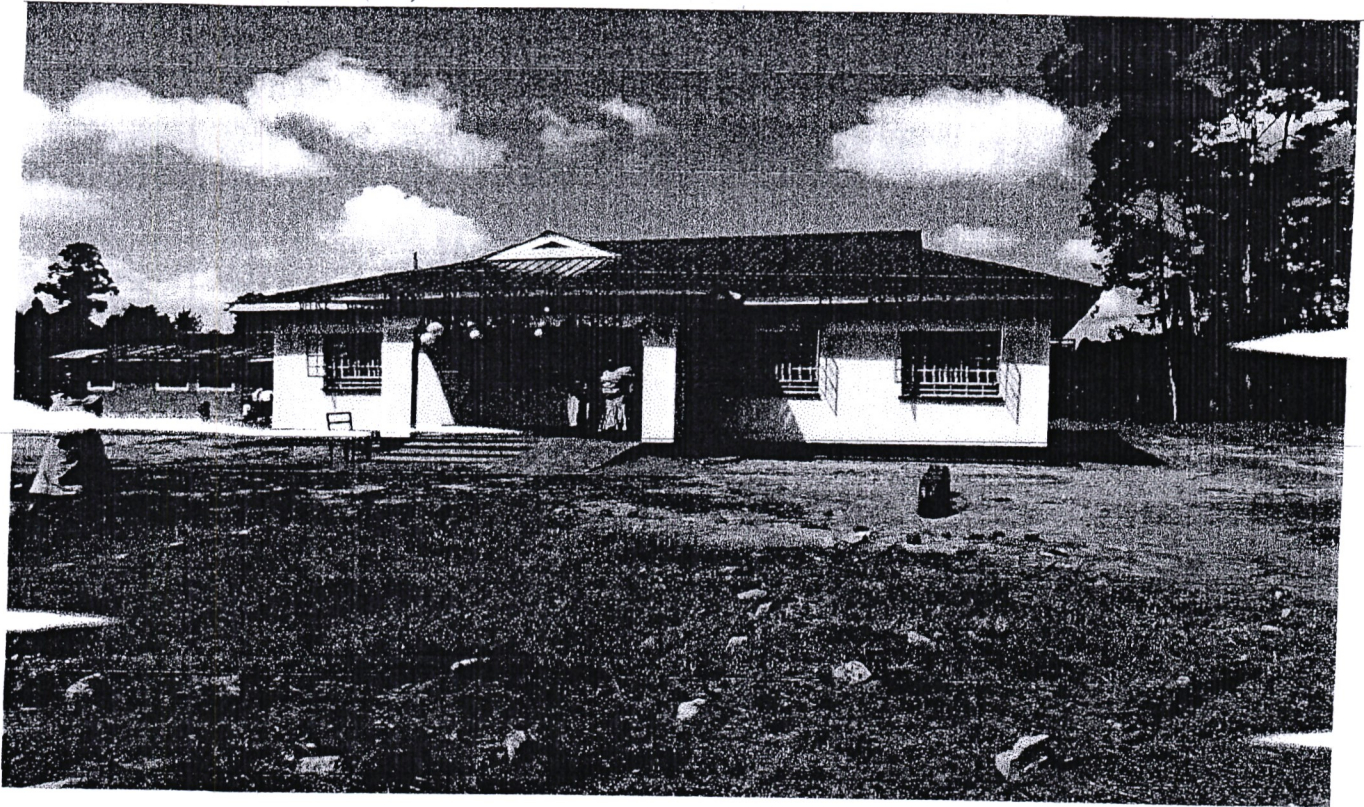
Kakoyi Primary School construction of Administration Block funded by Malava NGCDF Financial Year 2018/2019 and 2019/2020
