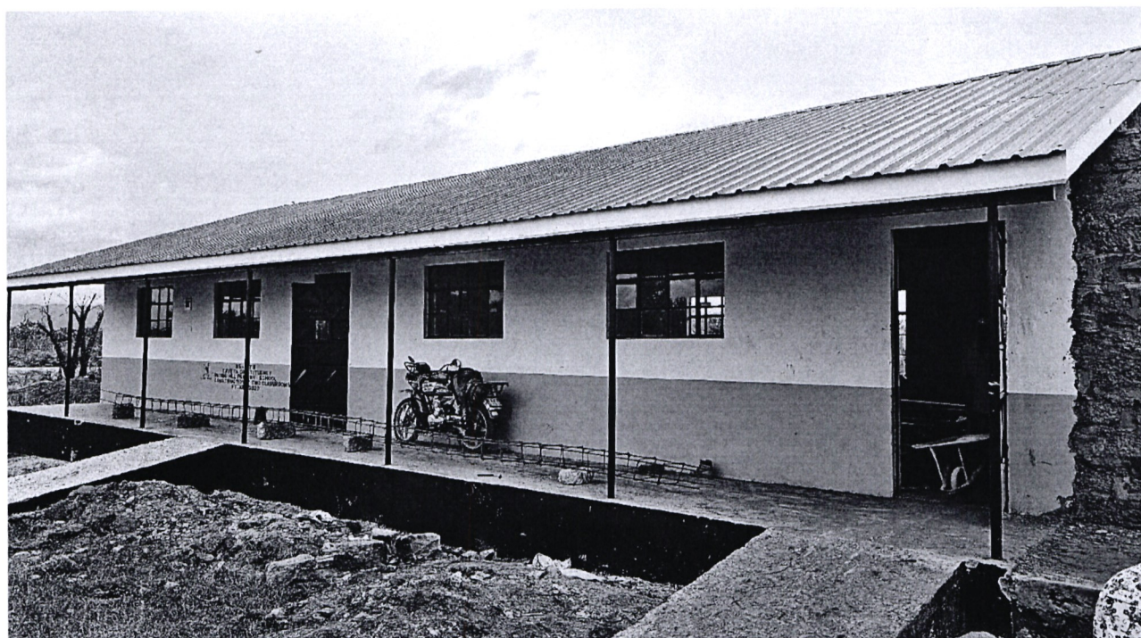
d. Construction of two complete classrooms at Patani Hill Primary School
