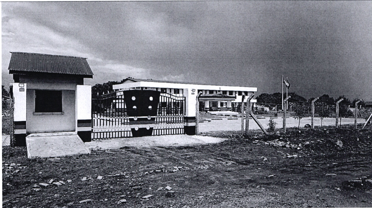
c. Completion of Taveta Sub-County Police Headquarters
