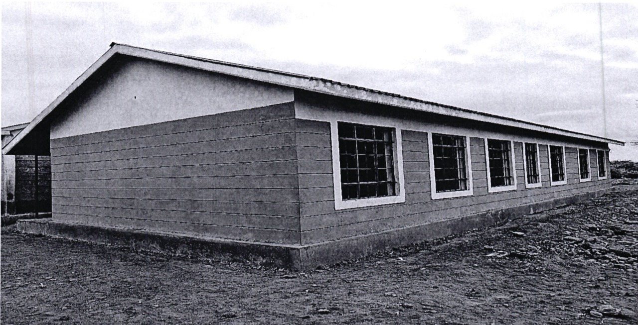
b. Construction of administration block – Abori primary school
