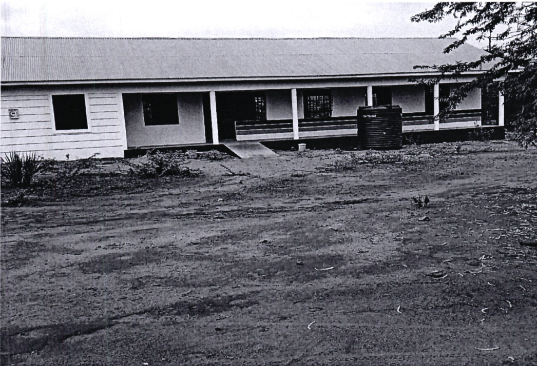
(f) Construction of Mata Chiefs Office
