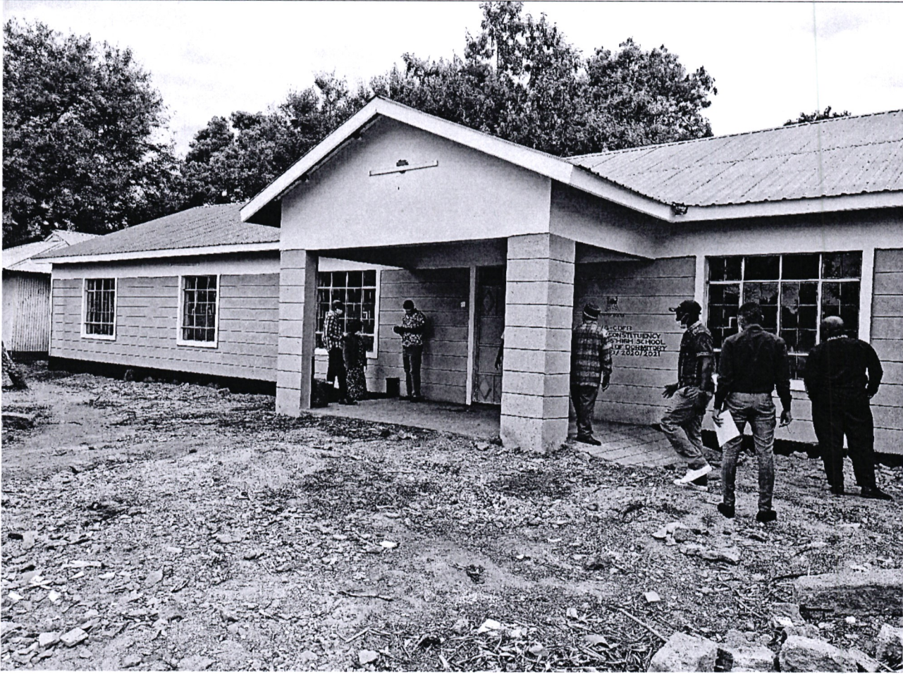
a. Construction of Boys Dormitory at Timbila Boys High School
