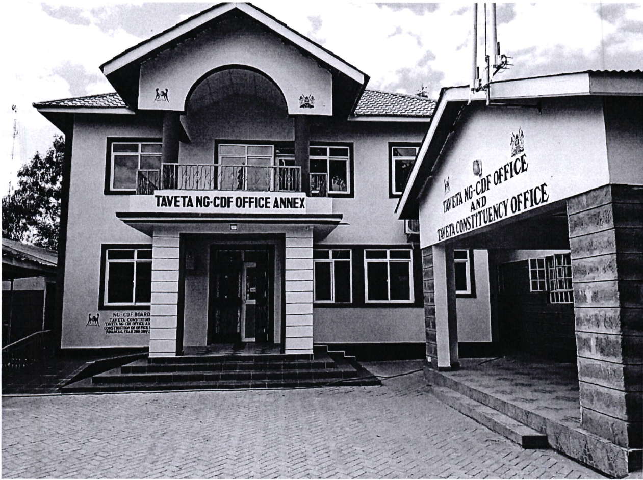
(i) Extension of NG-CDF Office- complete
