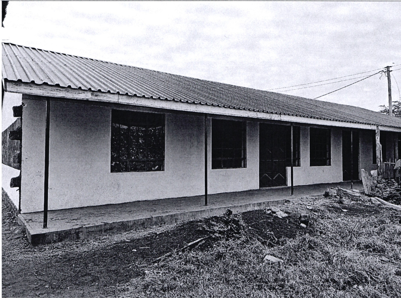
(j) Construction of classrooms – Sowene secondary school
