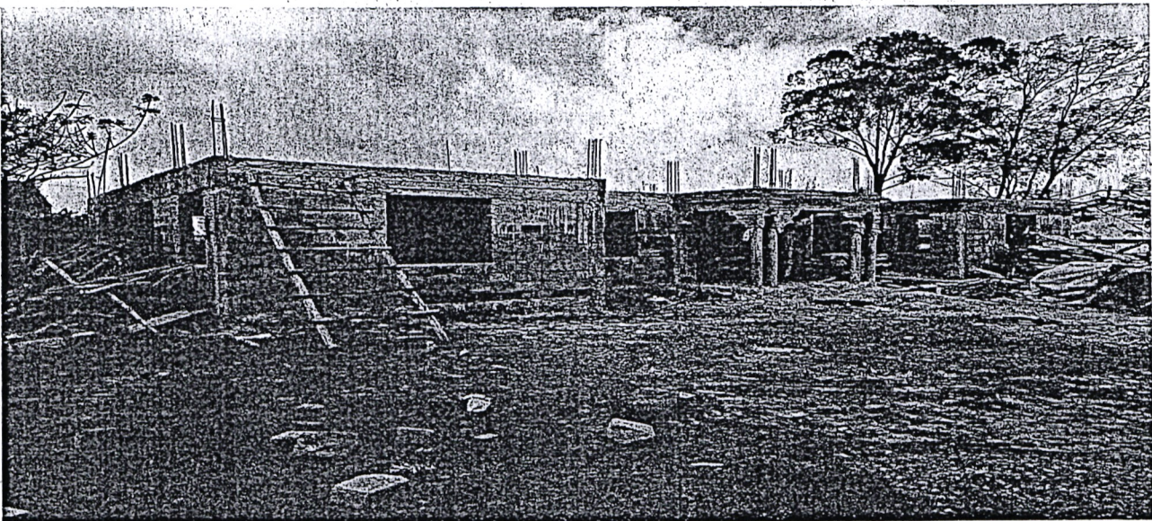
BIDII ASSISTANT COUNTY COMMISSIONER OFFICE-CONSTRUCTION OF ACC OFFICE- ON GOING
