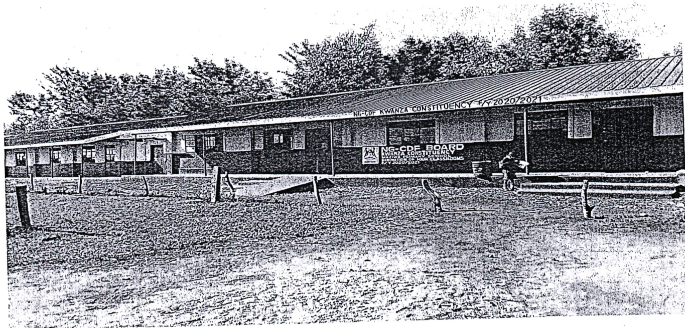
MAZIWA PRIMARY SCHOOL-RENOVATION OF FOUR CLASSROOMS-COMPLETE.
