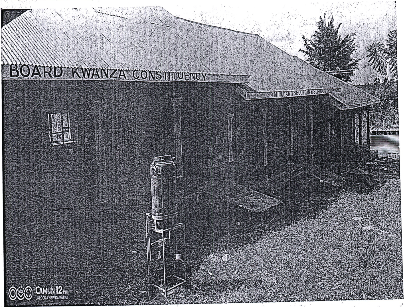
MILIMANI SECONDARY SCHOOL-CONSTRUCTION OF TWIN LABORATORY-COMPLETE.
