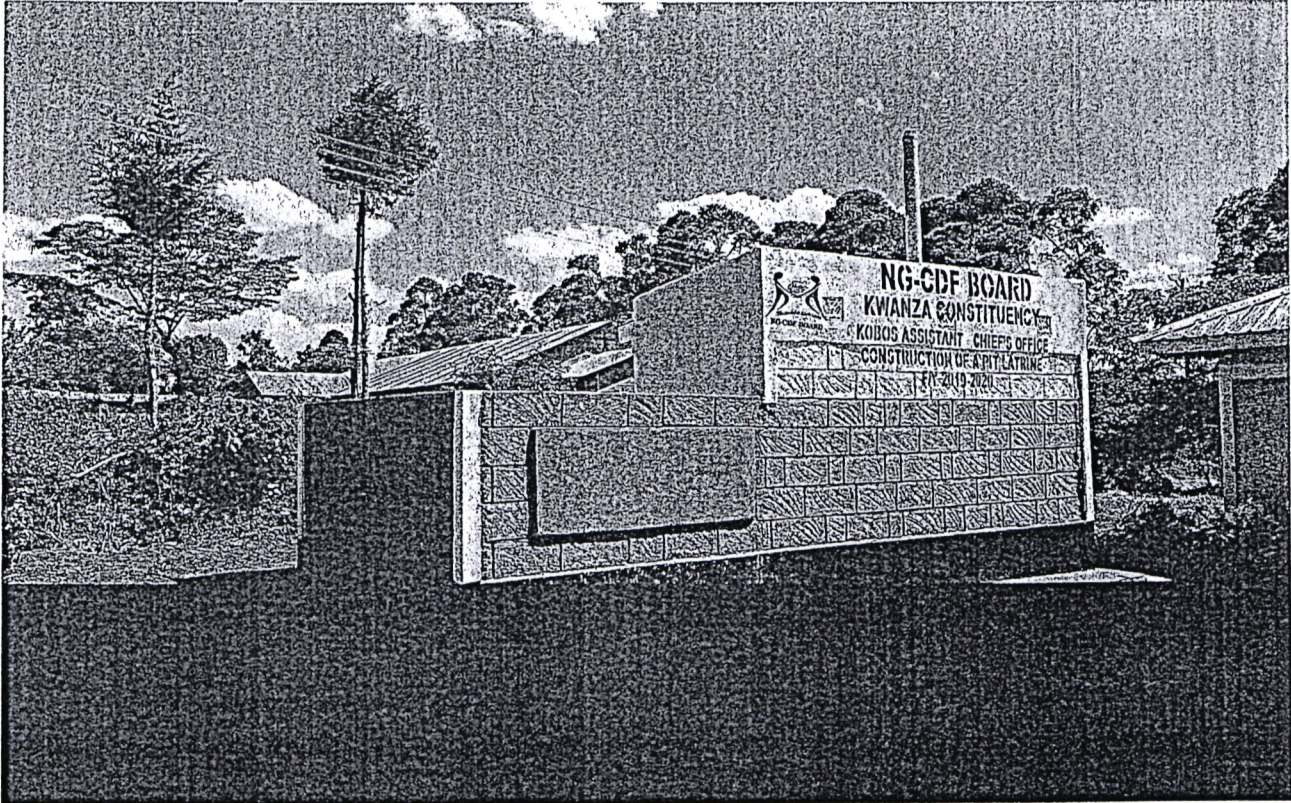
KOBOS ASSISTANT CHIEFS OFFICE- CONSTRUCTION OF PIT LATRINE-COMPLETED
