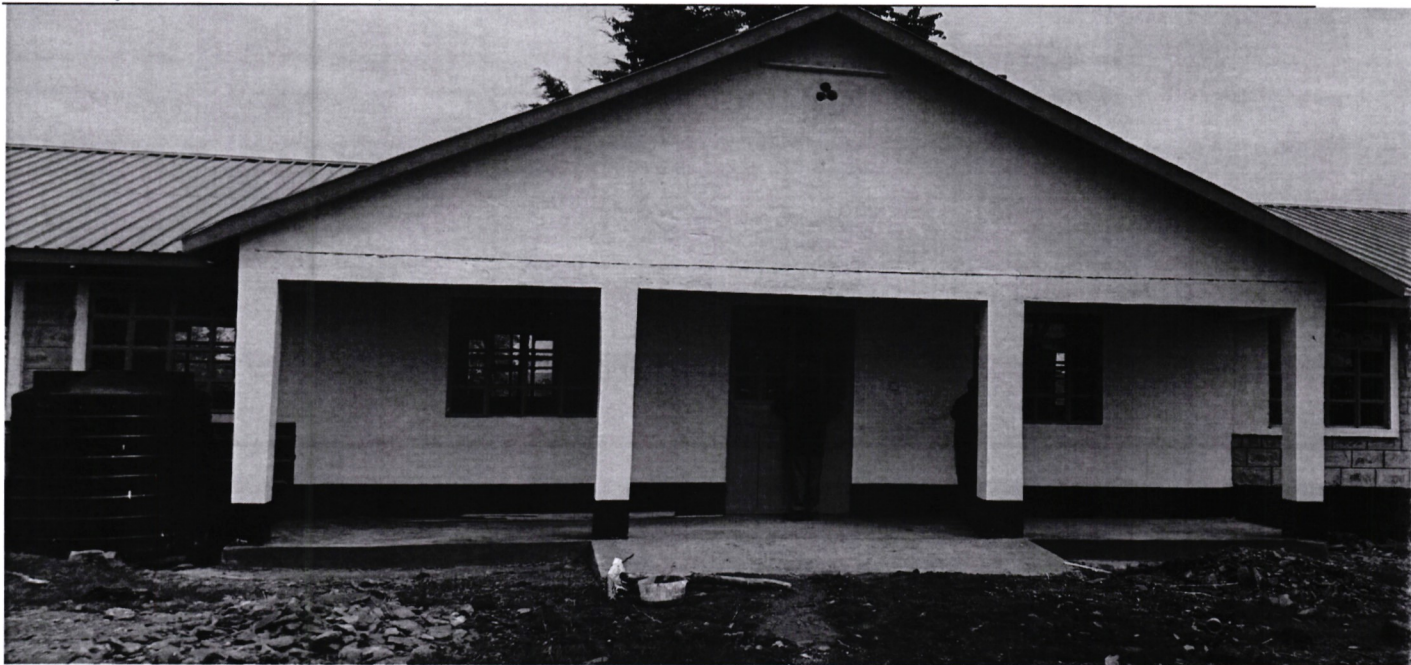
FIG 1.3: Saniak Secondary school: 120-capacity Boys Dormitory in final stages of completion. This will increase capacity of students being accommodated in the school
