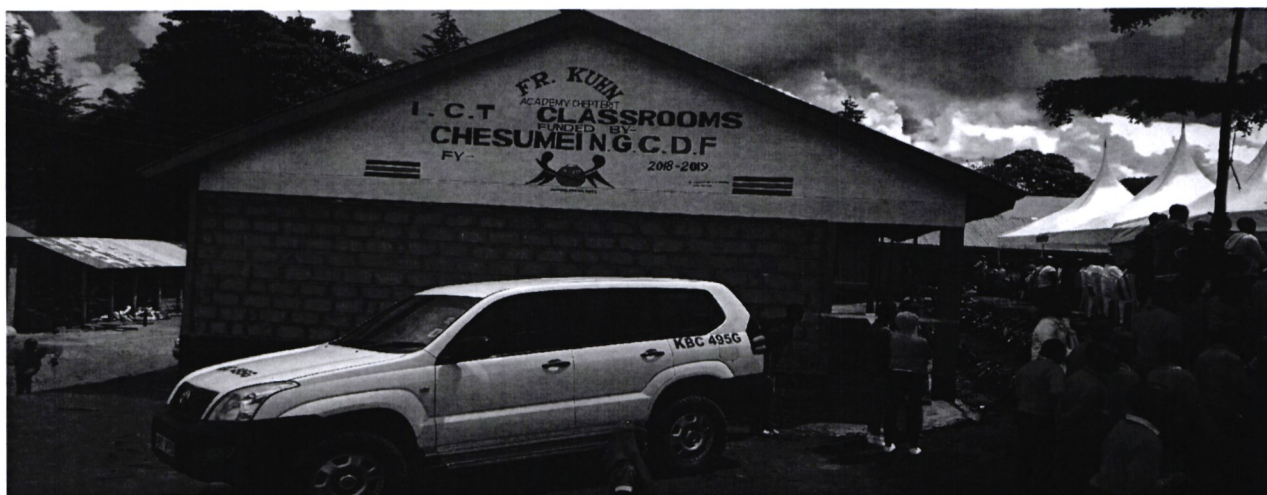
FIG 1.2 Fr. Kuhn Academy-Chepterit : Construction to completion of 2 ICT classrooms (FY 2018/19) to improve learning environment
