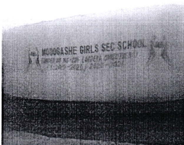
CONCRETE FENCE AT MODOGASHE GIRLS SECONDARY SCHOOL
