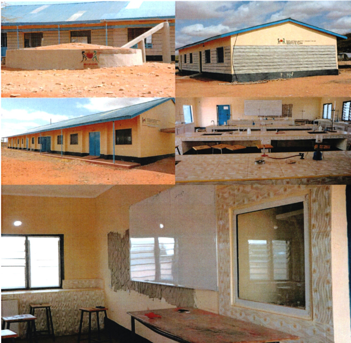
A well-equipped Modern twin Science Laboratory, two classrooms and an underground water tank with gutters for rain harvesting at Makaror Mixed Day Secondary School implemented by NGCDF Wajir West during the FY 2020/2021.
