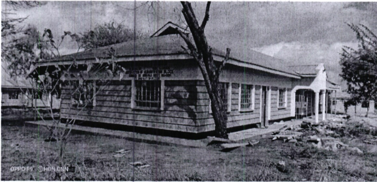
FIG 1.2: Administration block constructed at Kavaini Secondary School, completed FY 2019/2020 to improve teaching staff welfare.
