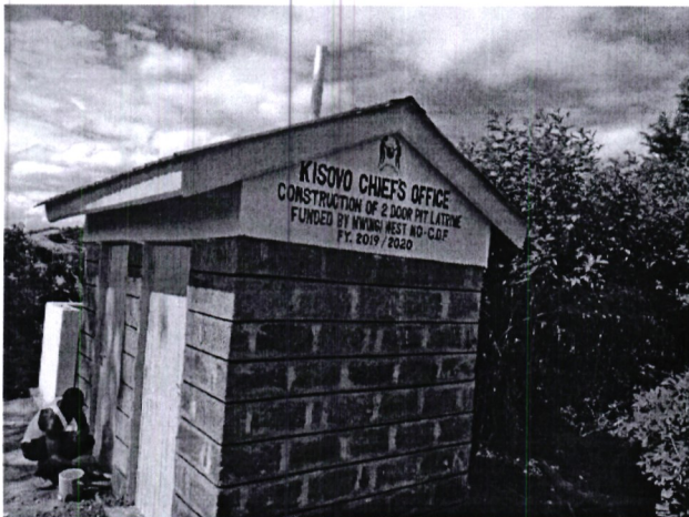
FIG 1.3: Constructed 2 door pit latrine at Kisovo Chiefs Office FY 2019/2020, to improve sanitation and working environment to the officers.
