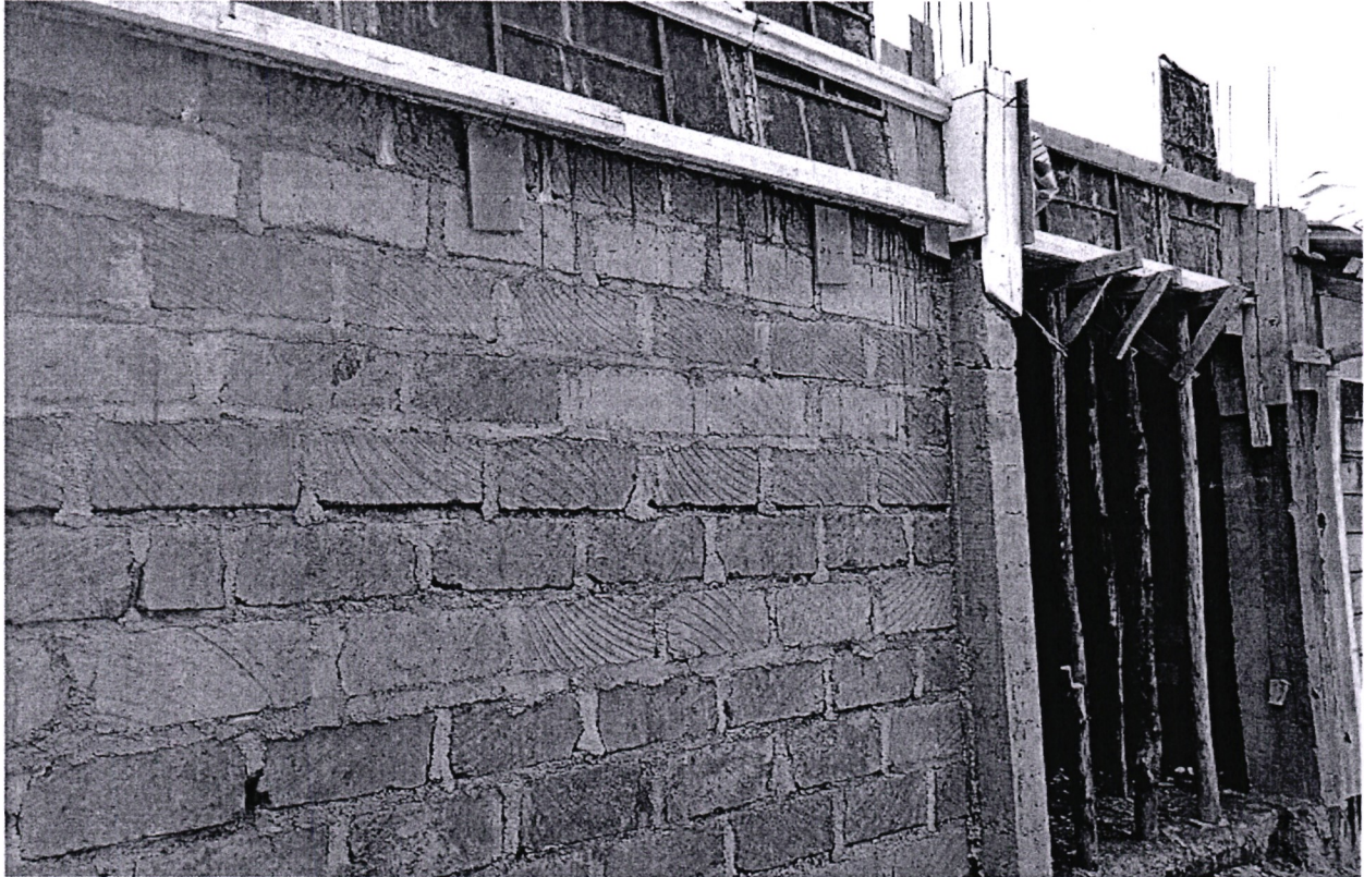
Figure 4. On-going construction of a twin laboratory at Kimathi secondary school.
