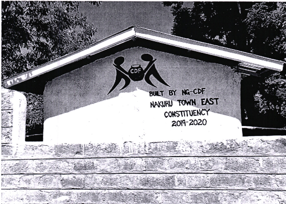
Figure 1. Bondeni primary school construction of 3 door toilet under environment vote complete.
