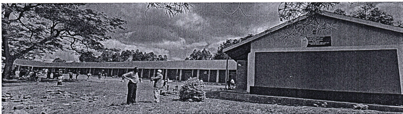
Fig 2 a : Atela Primary School: Rehabilitation of 14 Classrooms
