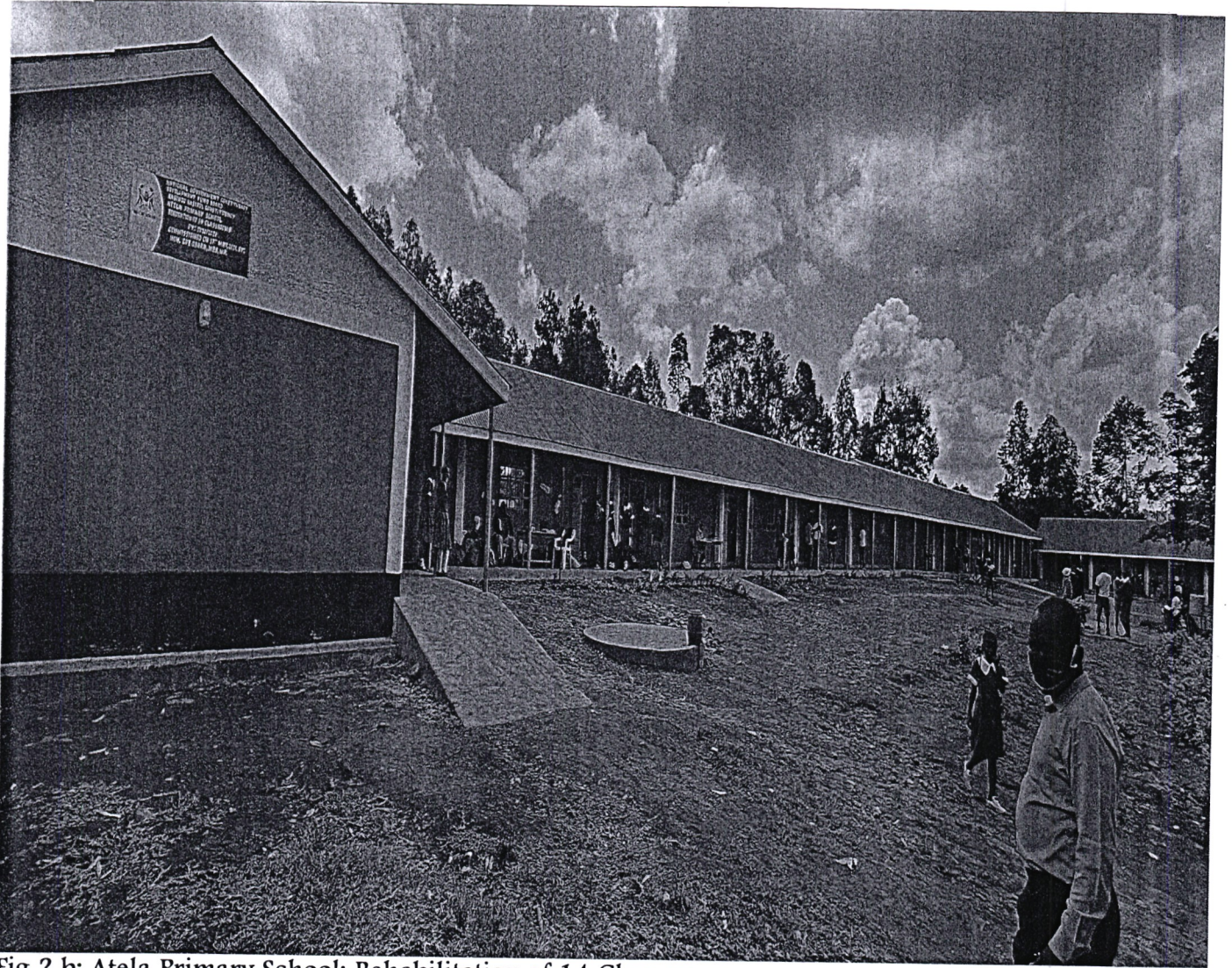
Fig 2 b: Atela Primary School: Rehabilitation of 14 Classrooms
