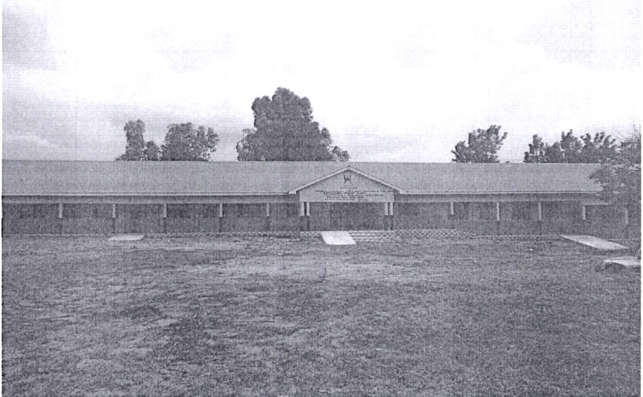
Figure 1: Katelynyang Primary school. -Finished four classrooms and Admin Block
