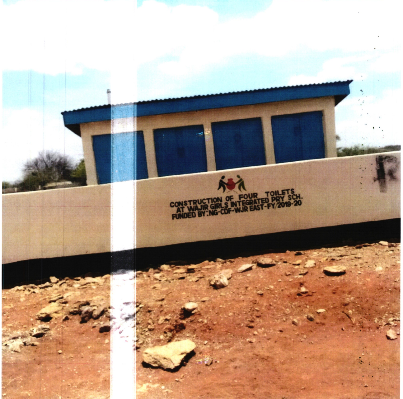
The construction of four toilets with septic tank at Wajir Girls Primary School Financial Year 2019/2020.
