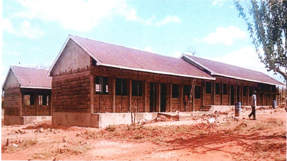
KMTC Tseikuru being under construction
