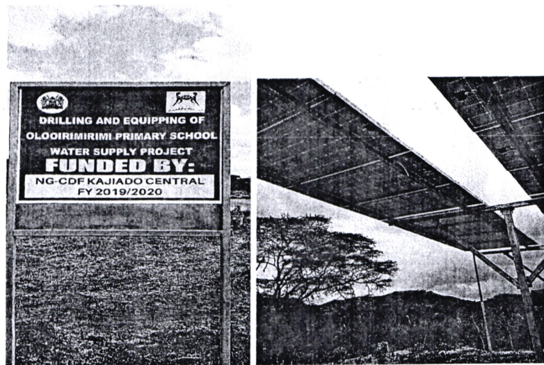
fig 1. Borehole equipping at oloirimirimi primary school
