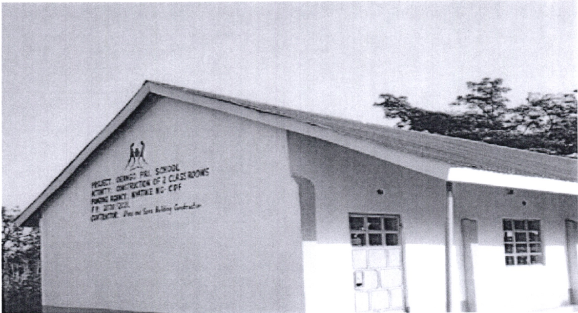
Construction of 2 classrooms at Orango Primary school
