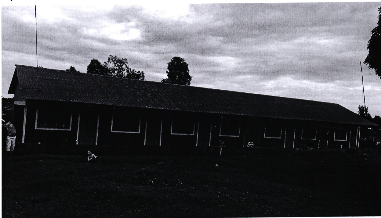
KITUTU CHACHE SOUTH NG CDF PROJECT-7 UNITS OF STAFF HOUSES CONSTRUCTED BY NG-CDF AT RUGA AP. LINE
