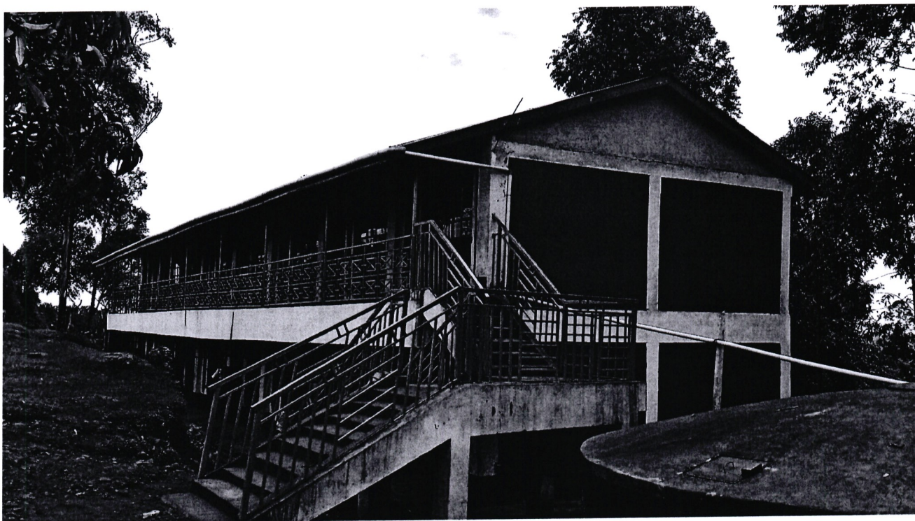
KITUTU CHACHE SOUTH NG CDF PROJECT-8 CLASSROOMS CONSTRUCTED BY NG-CDF AT KIANYABINGE PRIMARY SCHOOL
