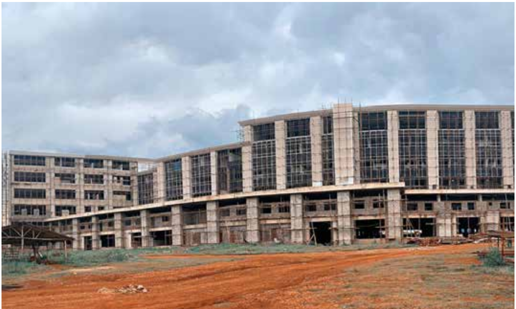
Kakamega Referral Hospital under construction 2019
