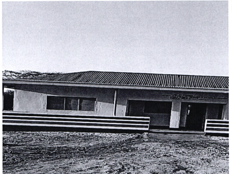
Mogilla Chiefs Office Nanam Ward Construction Of chiefs office to improve on provision of services to the citizens.
