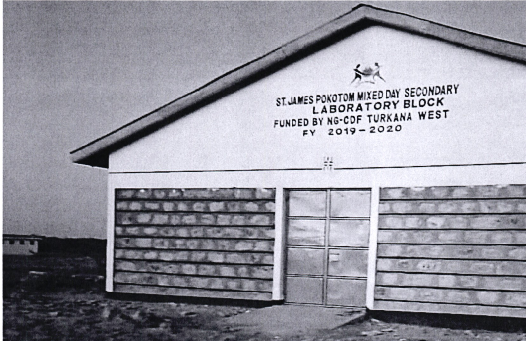
Pokotom Secondary School Kakuma Ward Construction of school laboratory
