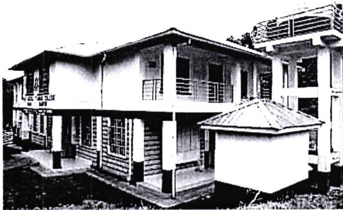
Administration block and Library at KMTC Maua Campus
