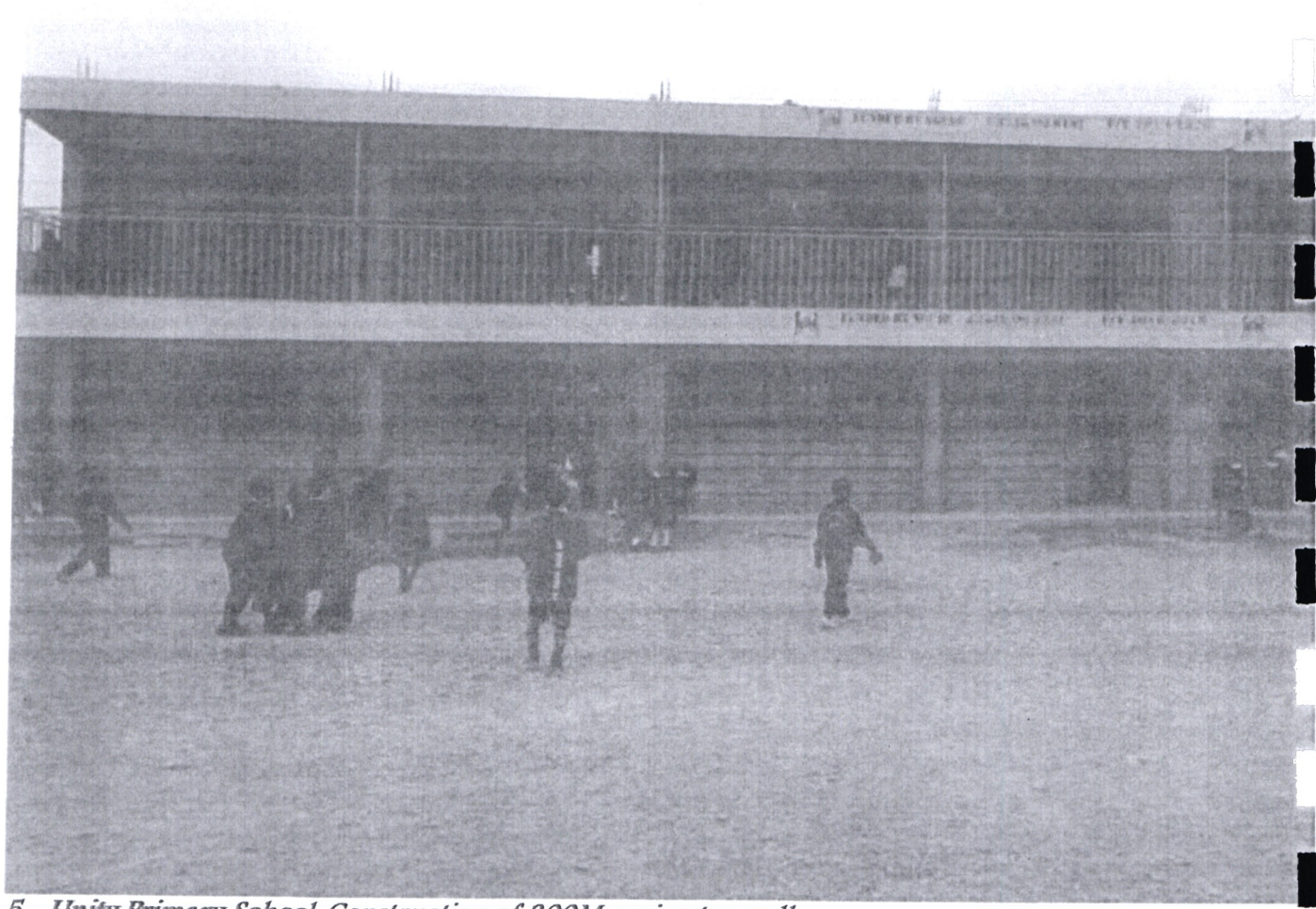
5. Unity Primary School-Construction of 200M perimeter wall
