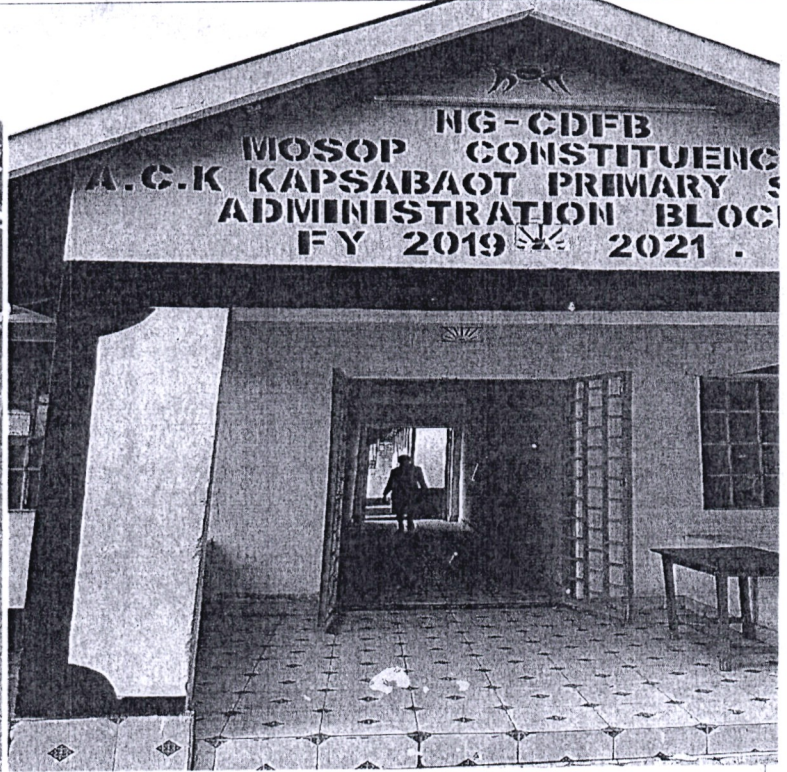
Kapsaboat Primary School ; Construction of Administration Block.
