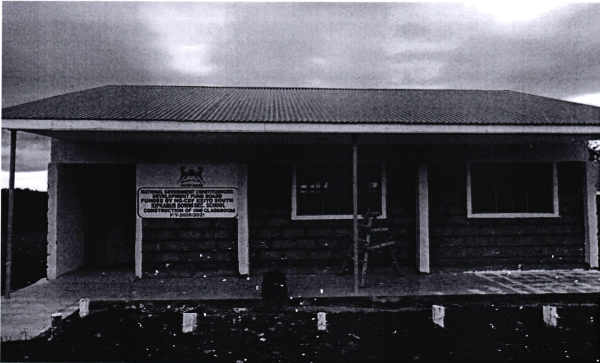
Kipkabus Downs Secondary School -Construction of one classroom
