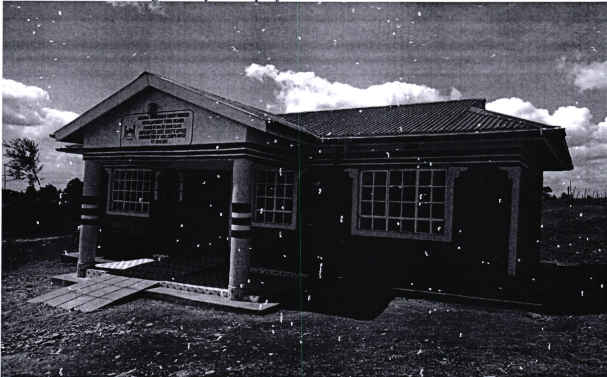
Kapcheptek Assistant Chief Office-Construction of Assistant chief office
