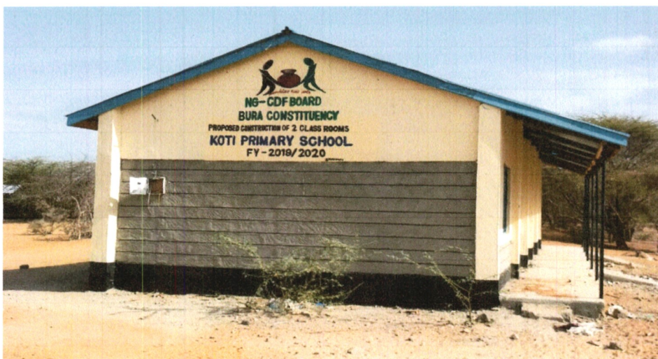
b) Construction of 2 No. classrooms at Koti primary school.
