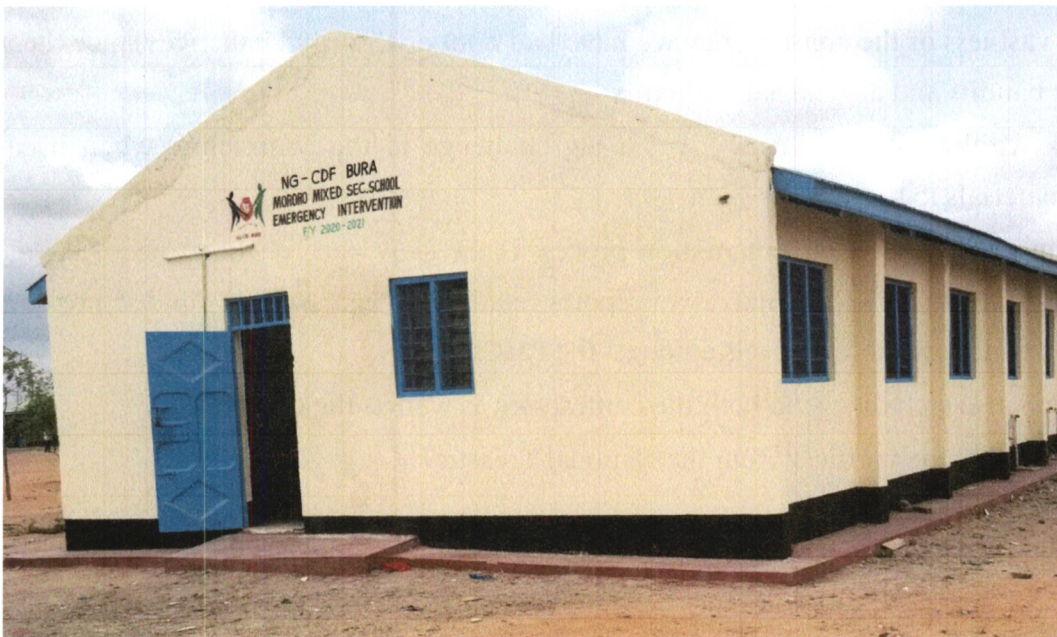
a) Emergency intervention at Mororo Mixed day secondary school.
