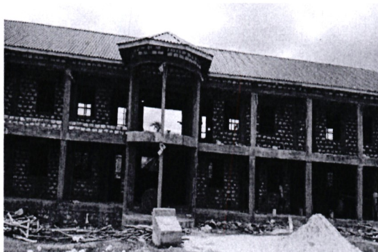
On-going construction at Kizurini Primary
