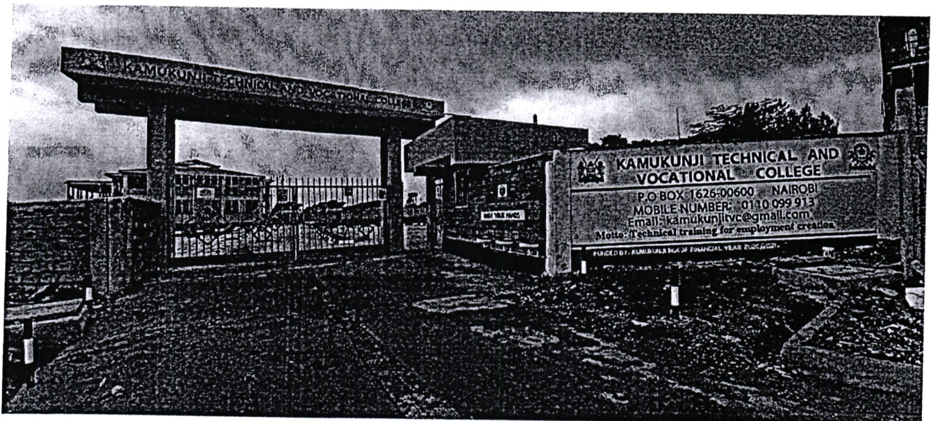
Completion of Kamukunji Technical and Vocational College
