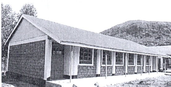
Kakrigu Mfangano Primary School (Construction of 3 classrooms)
