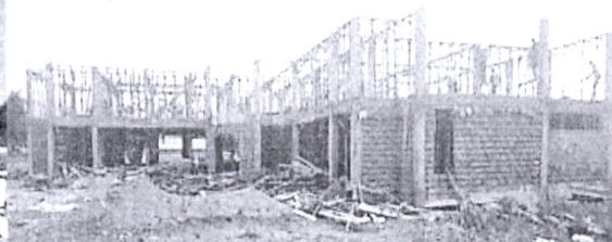
Mbita Medical Training College (Construction of administration block And lecture halls)
