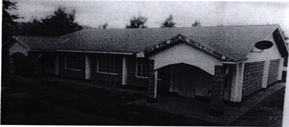
Fig. 1.1: Malaa Secondary School. Construction of Dinning Hall
