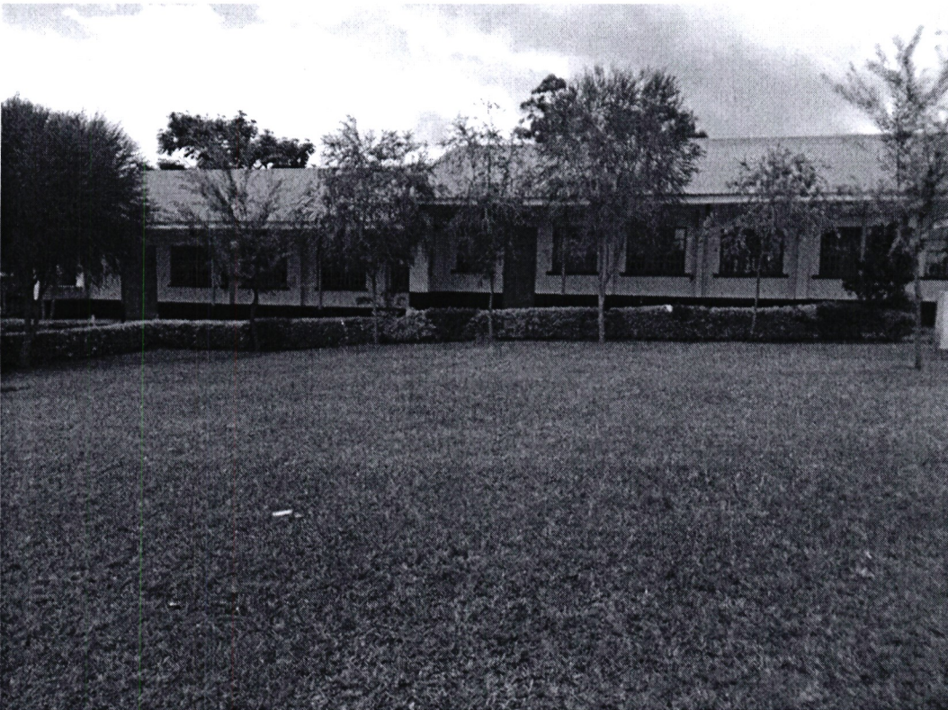
Pic. 3: Construction of Twin Laboratory at Kivagala Secondary School funded by Sabatia NG-CDF
