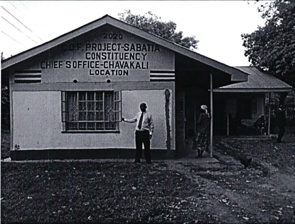
Pic. 2: Construction of Chiefs Office - Chavakali Location funded by Sabatia NG-CDF
