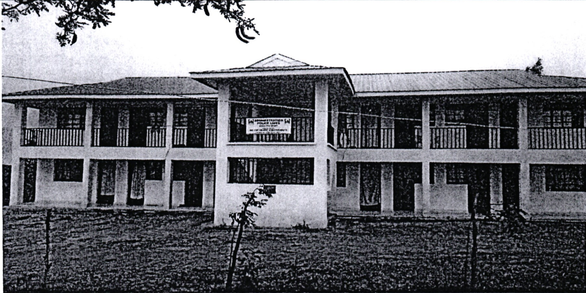
Image: Mukaa AP Camp Housing Project (Completion Date 30/6/2018)
