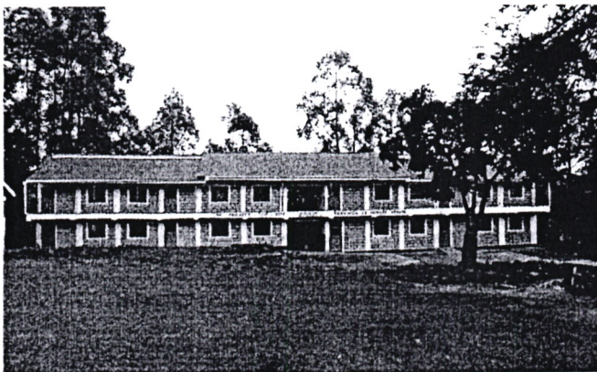
Eregi Mixed Primary School-Construction of 8No. Storey Classrooms
