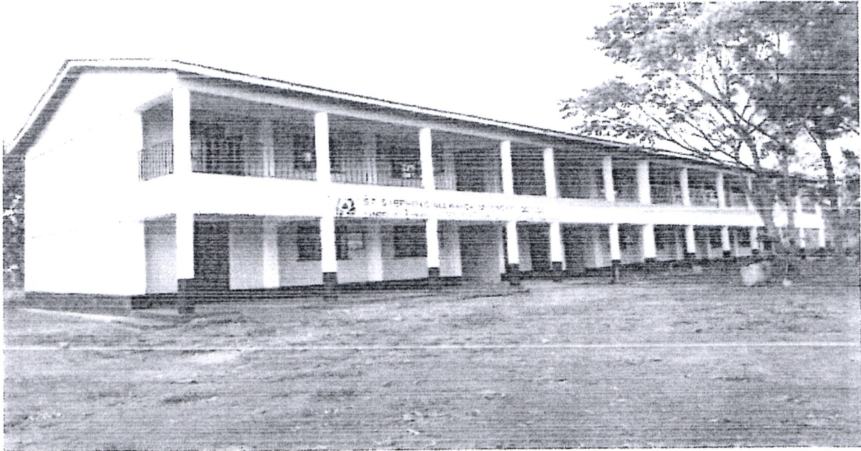
St. Stephen's Mulwanda Secondary School - Construction of a storey building comprising 4no.classrooms and a library. It is ready for use. It is located in Kisa Central Ward.
