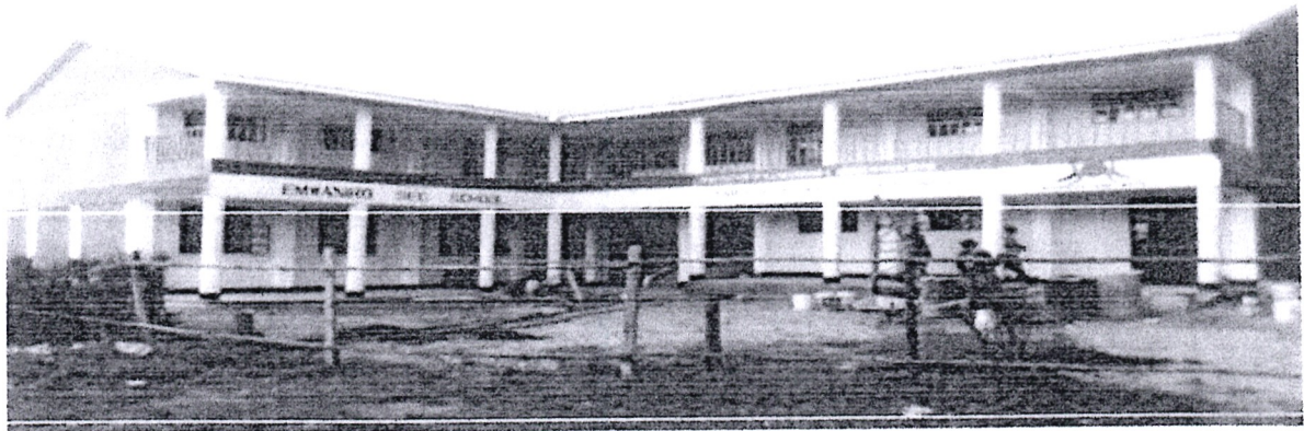
Emwaniro Secondary School - Construction of a storey building. Complete and handed over.
