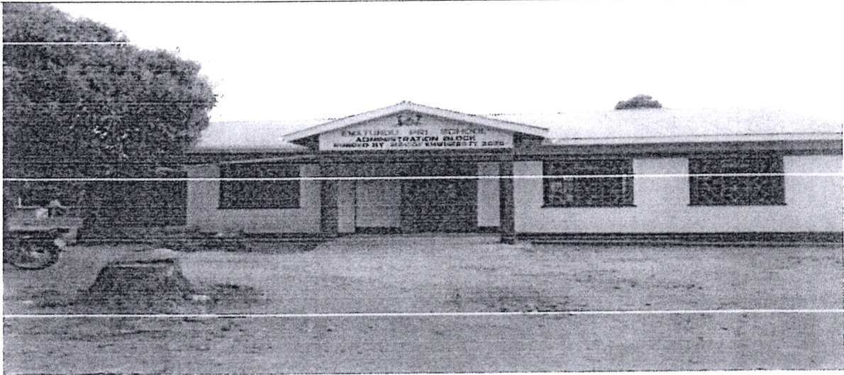
Ematundu Primary School - Construction of Administration block. Complete and ready for use/handover.
