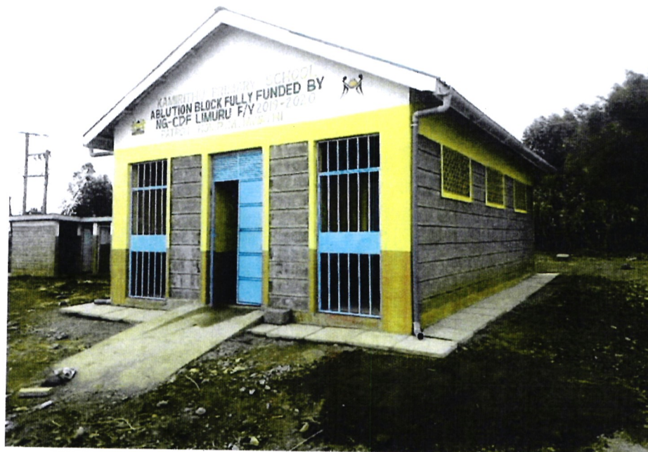
The modern Toilet Block.
