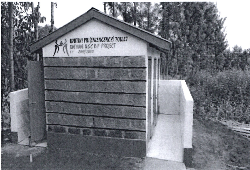
Fig. 4 Wutini Primary school- 6 door toilets
