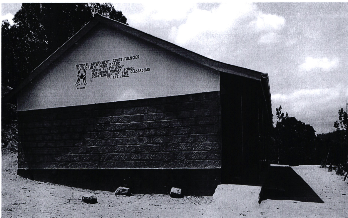
Figure 1.2 Matondoni Primary School-Construction of 2 No. Classrooms
