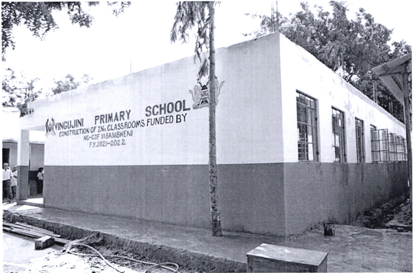
Vingujini Primary School (Construction of 2no Classrooms)
