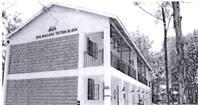
Construction Of Migori Primary School Classroom Of Ksh.5,000,000. Fy 2019/20/21
