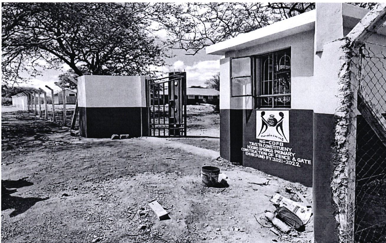
d. Fencing and Construction of gate at Njoro Springs Primary School
