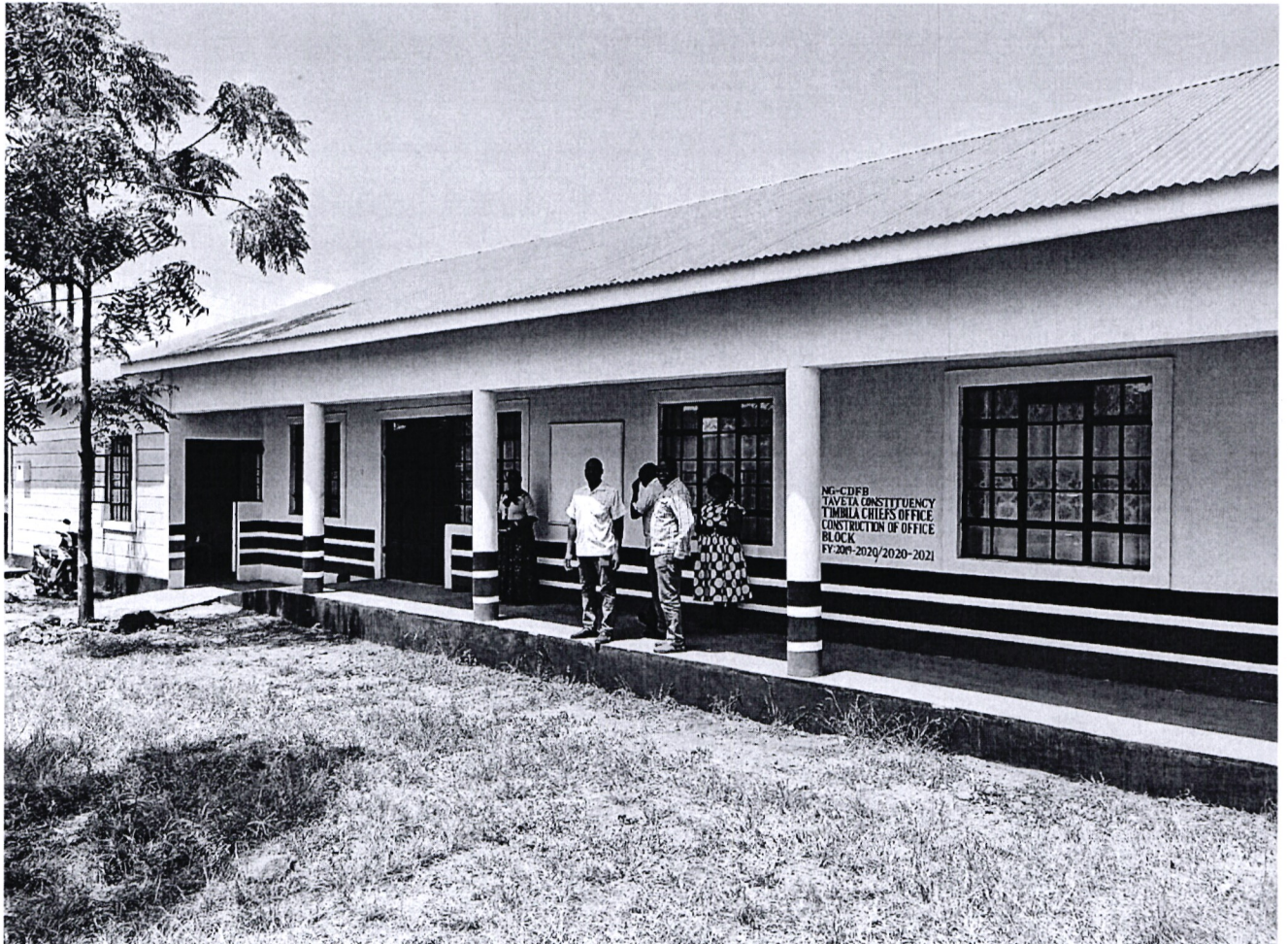
c. Construction of Timbila Chiefs Office
