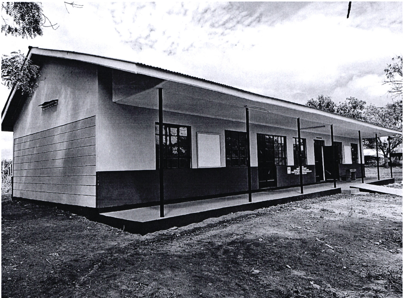
a. Construction of Two Classrooms at Msheghesheni Primary School
