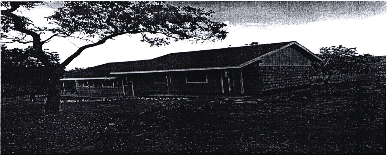
Kiptaiwa Primary School – Construction of Two Classrooms
