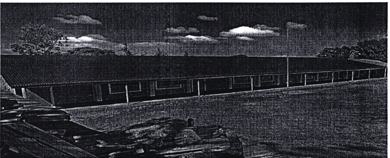
Kasesia Primary School – Construction of Four Classrooms
