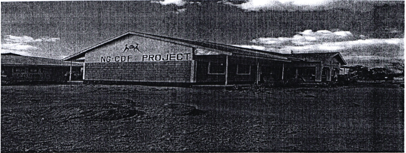
Barwessa Secondary School – Construction of Administration Block
