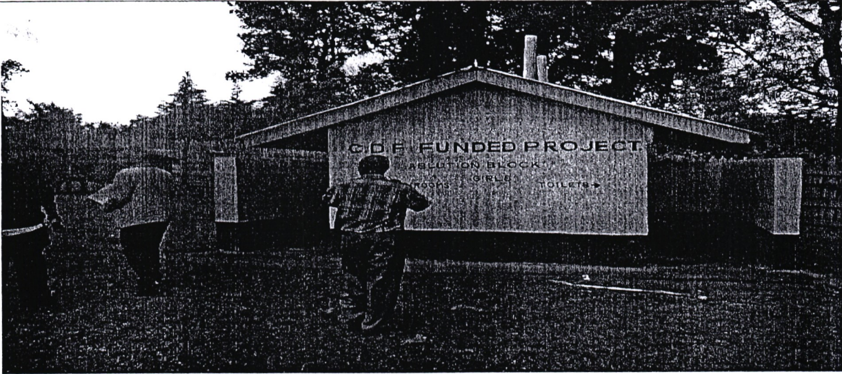
Ossien Primary School – Construction of Ablution Block
