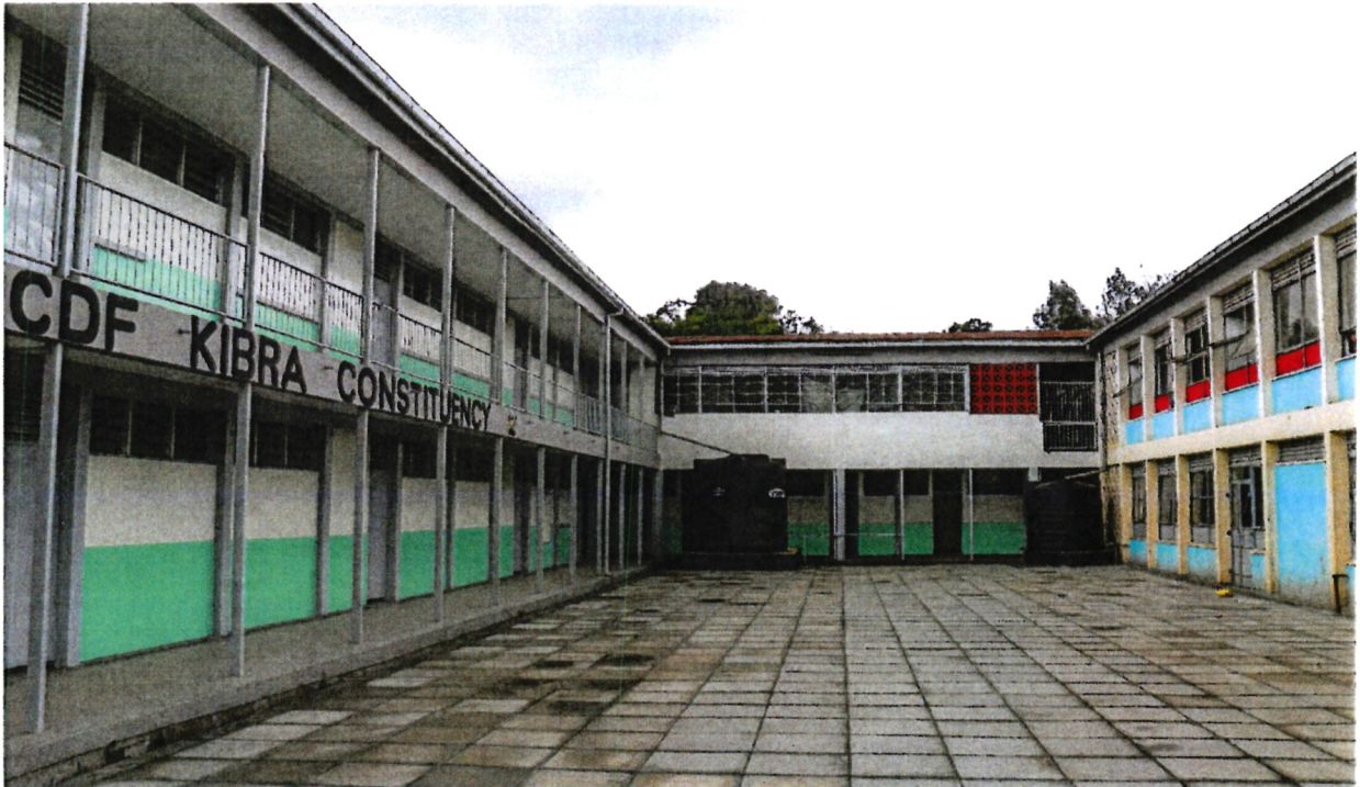
Rehabilitation of Toi Primary School.
