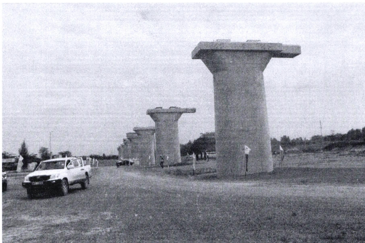
Picture 4: Construction of Athi River Super Bridge
