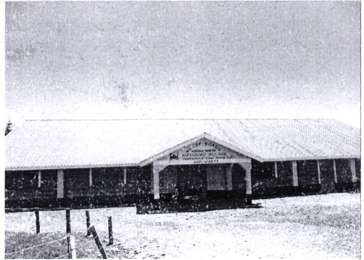
Kiptororo Secondary School-Construction of Dining Hall-Kiptororo Ward
