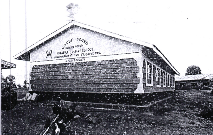
Kibaraa Pri School-Construction of 2 Classrooms-Kiptororo Ward
