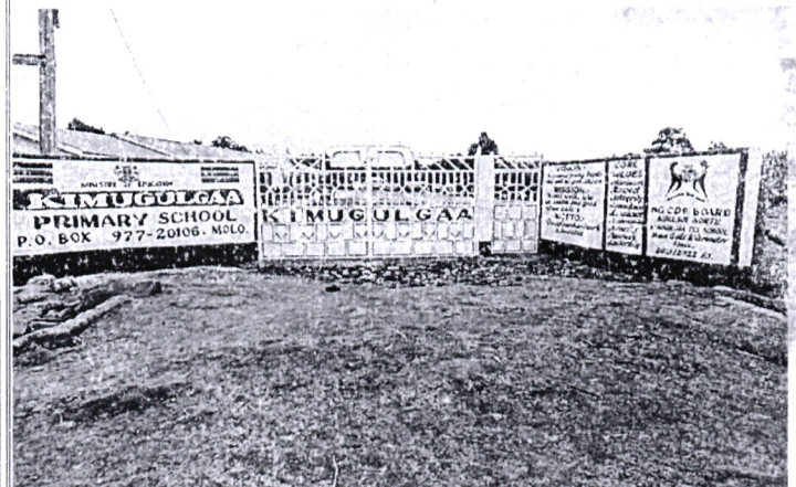
Kimugul Gaa Pri School-construction of Main Gate/Perimeter Fence-Kamara Ward
