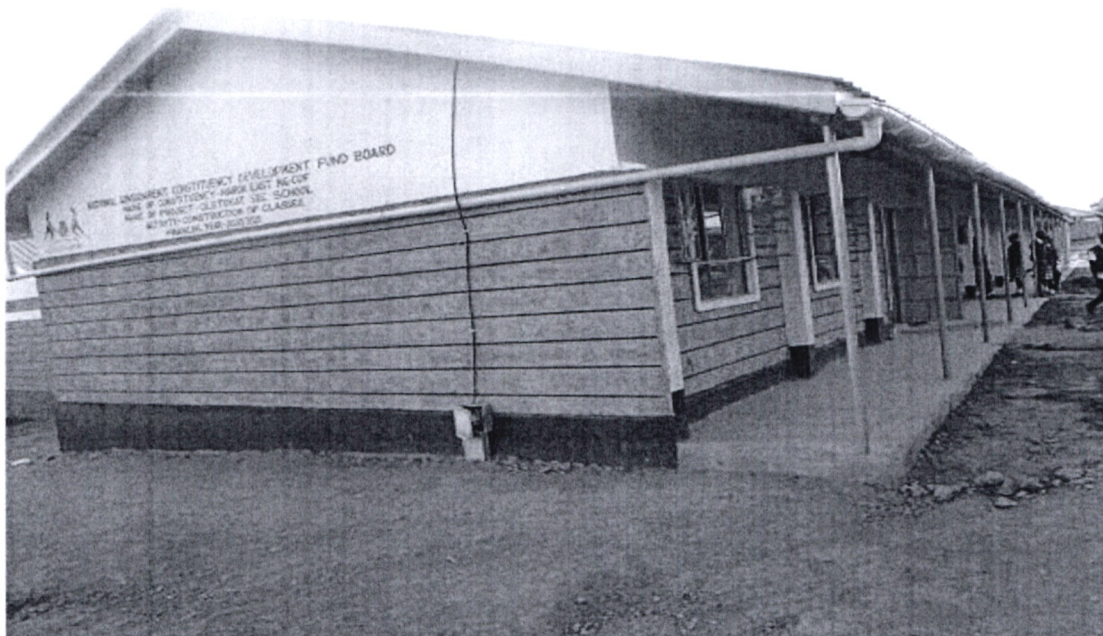
Oletukat Secondary School 3 No. Classrooms.
