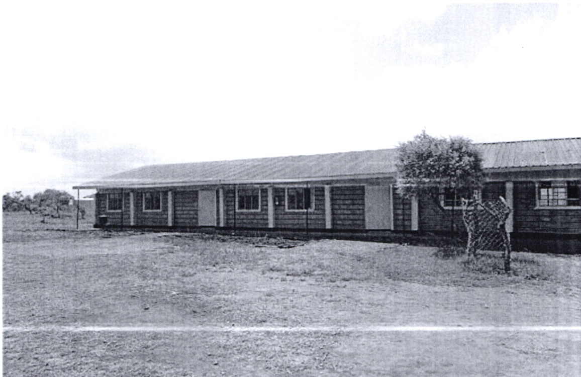
Olesharo Girls Secondary School Classrooms
