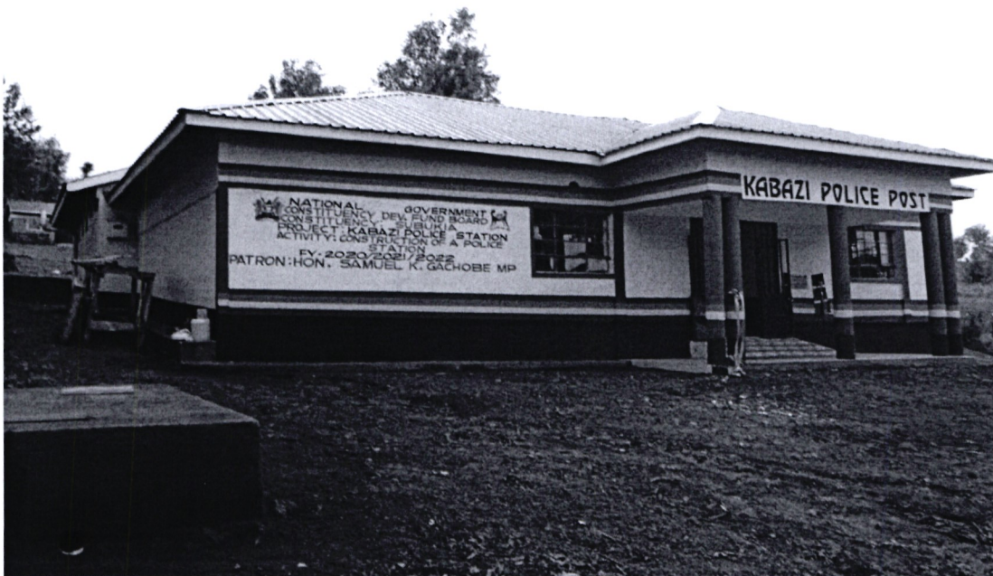
KABAZI POLICE POST- Construction of police post offices
