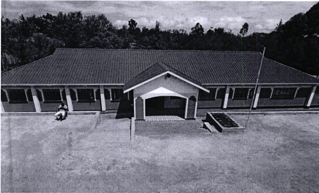
OLDONYO MARA SECONDARY-Construction of Administration block
