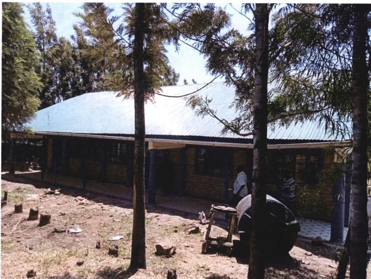
Figure 1: Completed Nyamasare Sec. Laboratory which has improved practical lessons to students
