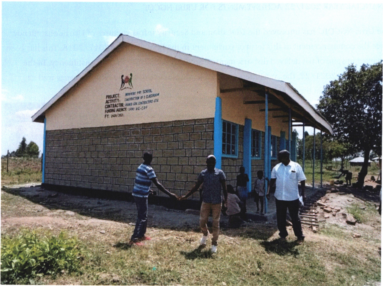
Figure 2: Completed Classroom at Minyere Secondary which has helped in 100% transition
