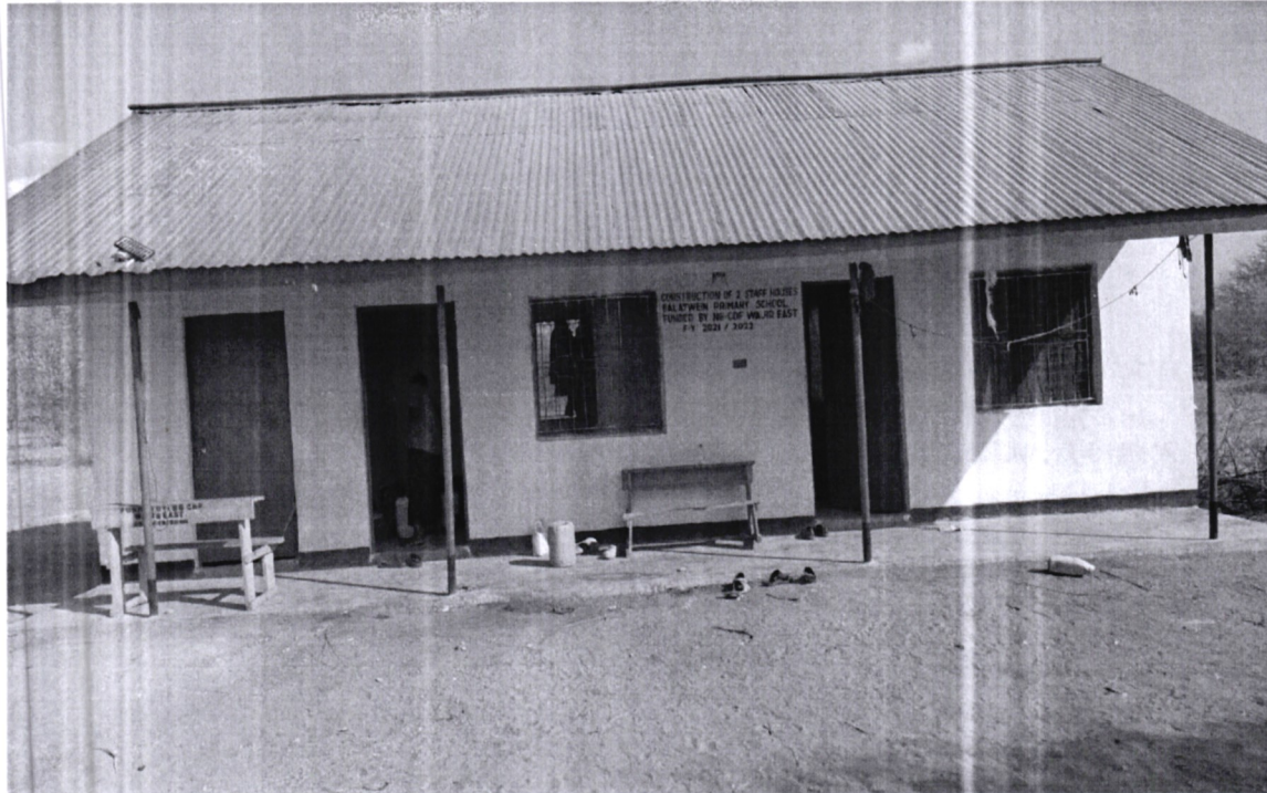
Balatwein primary school- construction of two staff quarters FY 2021/2022
