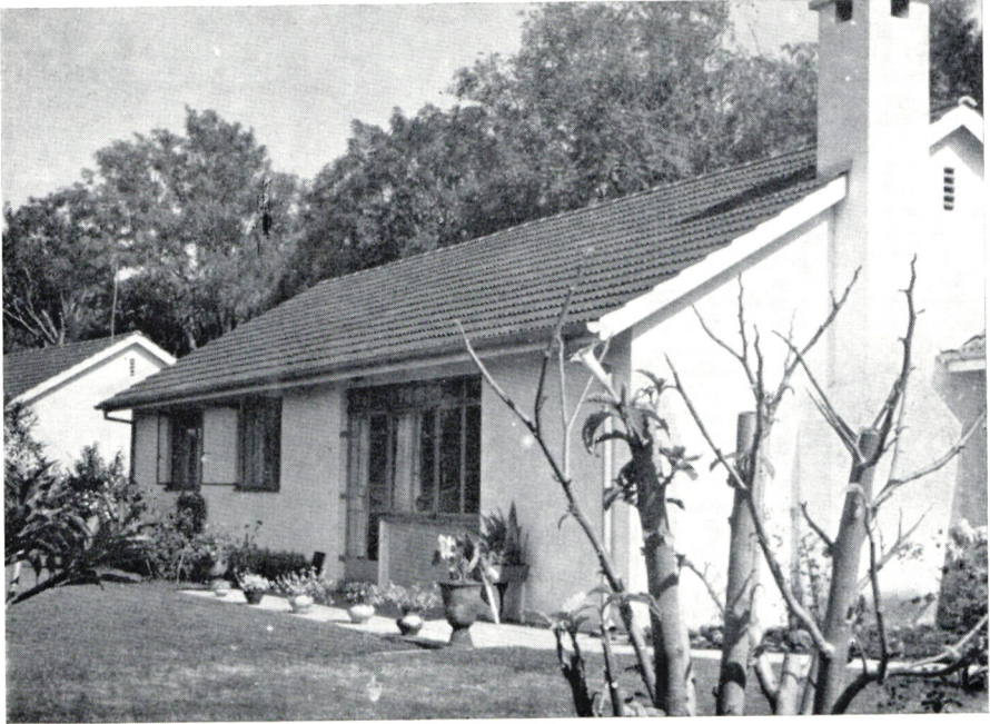
One of the newly constructed staff houses
